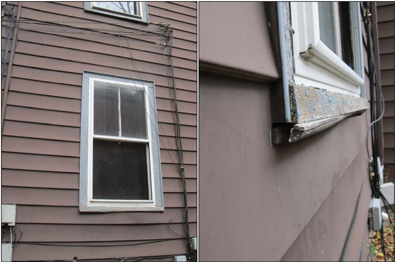
Aluminum siding showing the casing around the windows and condition of the remaining window casings.
